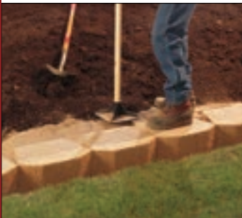
2. Place & Compact Backfill
